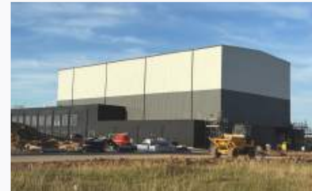
Bristow's new search and rescue training facility due for completion end 2025
