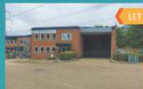
Woodside Industrial Estate, Eastleigh - Industrial Unit 5,339 sq ft
